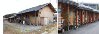
One innovative solution in Tohoku Fukushima Prefecture built more than 6700 wooden temporary houses (Temporary housing) + (wooden) + (local builders)
