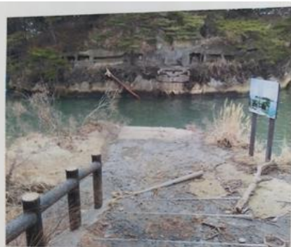
雄島に架かる「渡月橋」が津波により落下 Togetsukyo Bridge of Oshima Island washed away by th tsunami.
