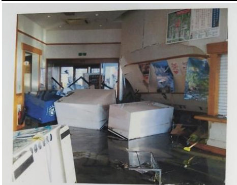
津波で自販機が流出し壁やドアを破壊(観光協会案内所窓口前) Inside the Rest House where the door and the vending machine were destroyed by the tsunami.
