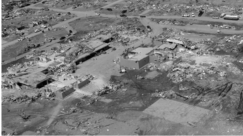
the damage to Plaza Towers Elementary School after an F5 tornado touched down in the Moore, Okla., area on May 20, 2013. Photo courtesy of Jocelyn Augustino/FEMA
